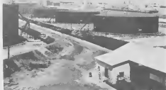
BLACK STORAGE tanks absorb the sun's rays as heat is needed to help heavy products such as crude oil flow through pipelines.
